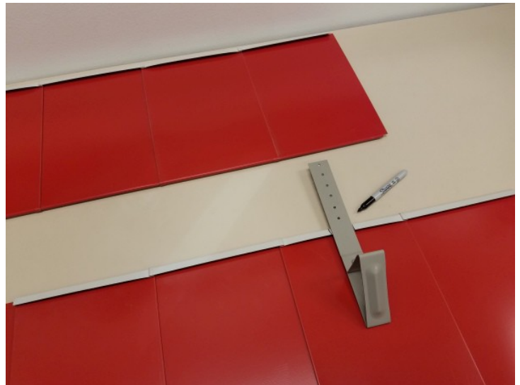
Mark the upper seam where the snow hook needs to be installed
