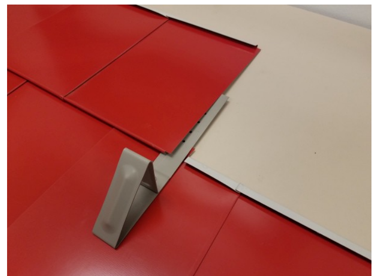
Snow hook can be placed under the vertical seam if needed
