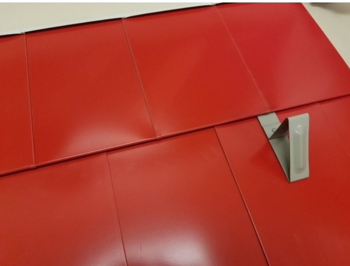
Interlock the next panel over the snow hook
